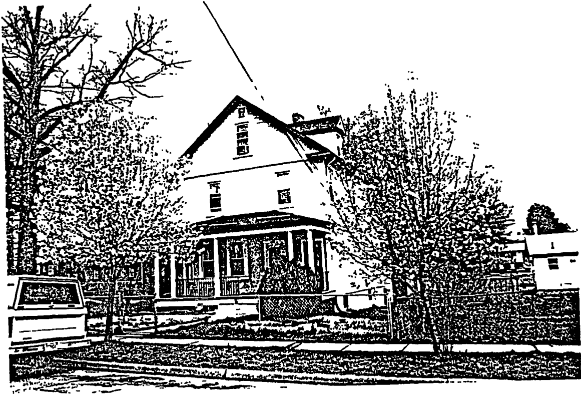
Front Gable at 4900 Queensbury Road
