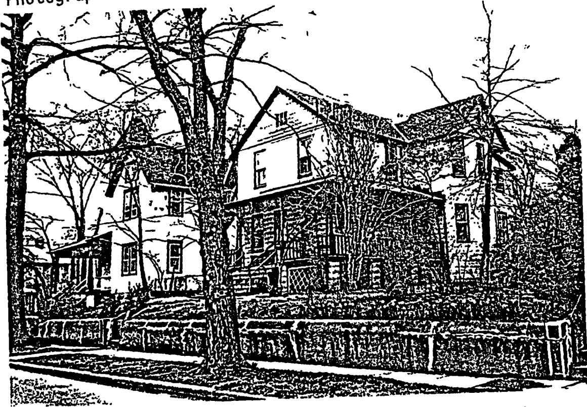
Cross Gables at 4606 and 4608 Queensbury Road
